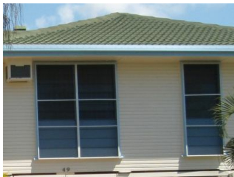
Figure SC6.2.3.17 Illustrates an example of a full height window, acceptable in 1960’s Defence Housing Precinct only
